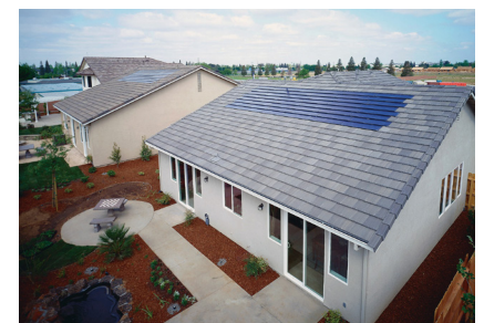
2.2 kW Residential BIPV System 10
