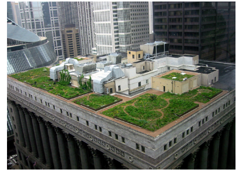
City Hall Green Roof, Chicago, Illinois 22
