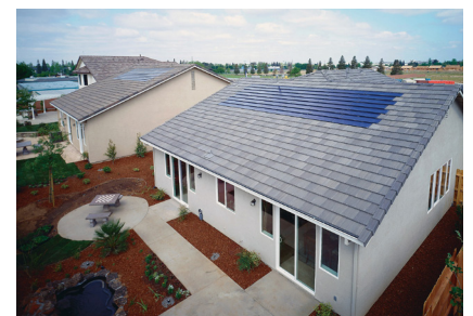
2.2 kW Residential BIPV System 13
